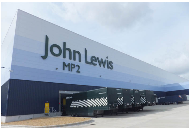
The 650,086 sq.ft John Lewis distribution centre at Magna Park, on the M1 motorway close to Milton Keynes.
