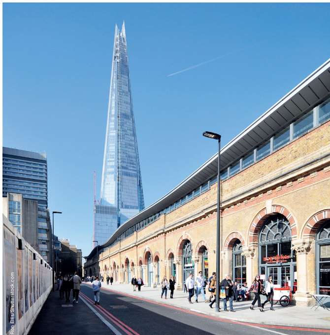
London Bridge Railway Arches
